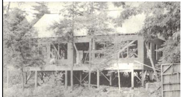
1948 Club House under construction on wooden piers
